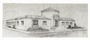
MODIFIED SPANISH architecture is the design for the new home of KTSM El Paso. Building will be of completely modern construction, with the latest innovations in acoustic design for the three studios. There is also special emphasis on modern lighting. Brick covered with cream colored stucco is to be used with, according to Karl Wyler, general manager, "the reddest tile roof we can possibly lay our hands on."
